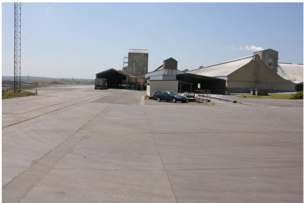
Photograph A.6 Shed 1, showing the railway line
